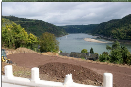
Construction site, 26 Sep-
