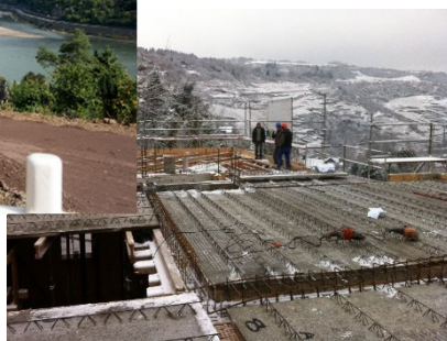
Construction work, as at 30 November 2010 (Photo: Herbert Steffen)
